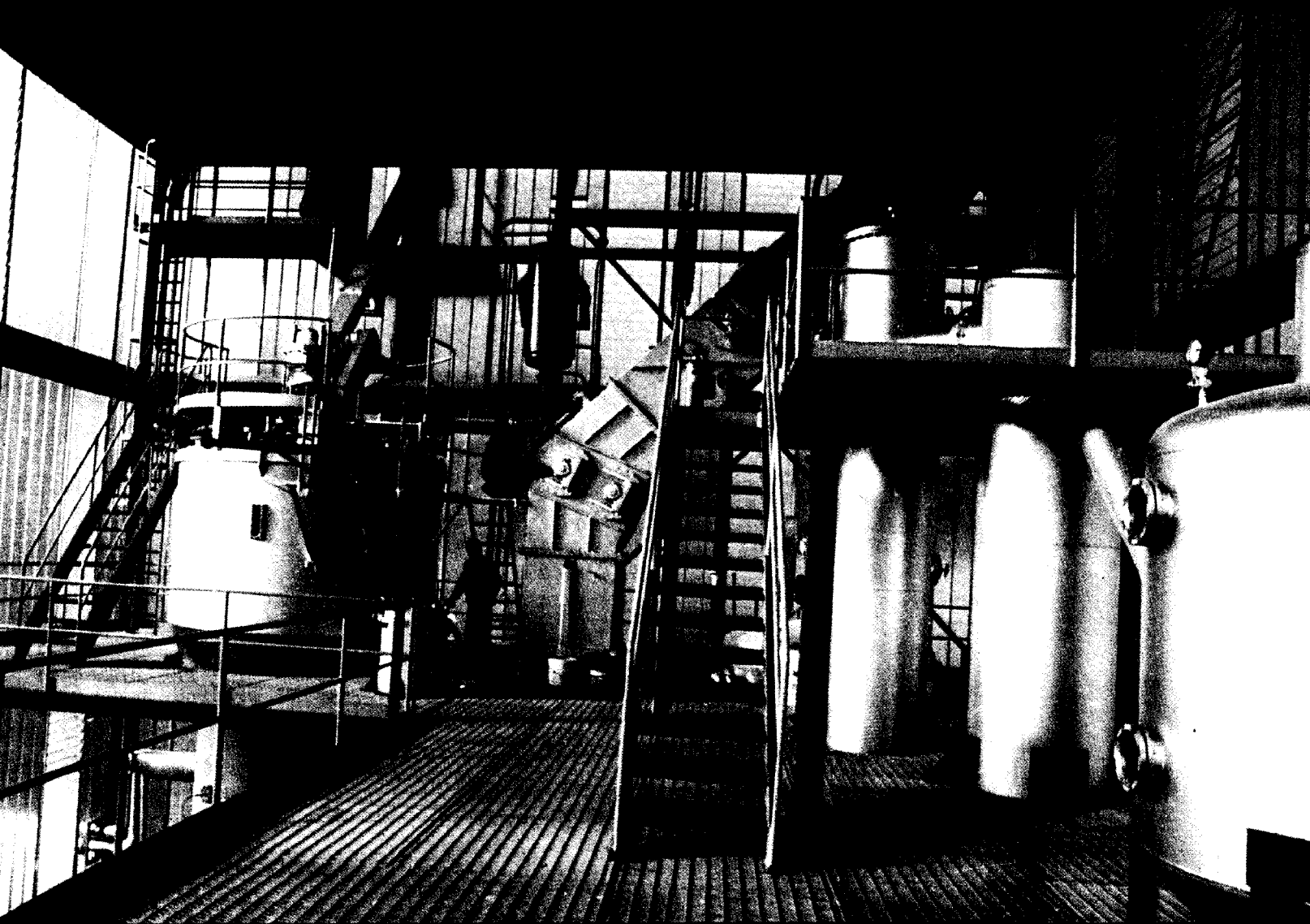
Detail of continuous solvent extraction plant in a turn-key factory
